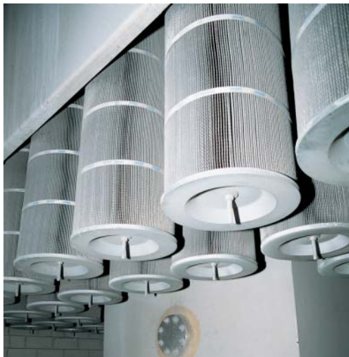
GTC surface-loading filter cartridges at a chemical plant in Germany
