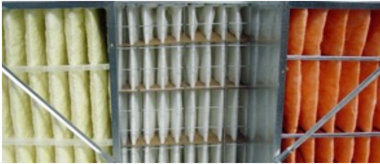
Plastic, Cardboard and Metal (l to r) Finger Media Separators
